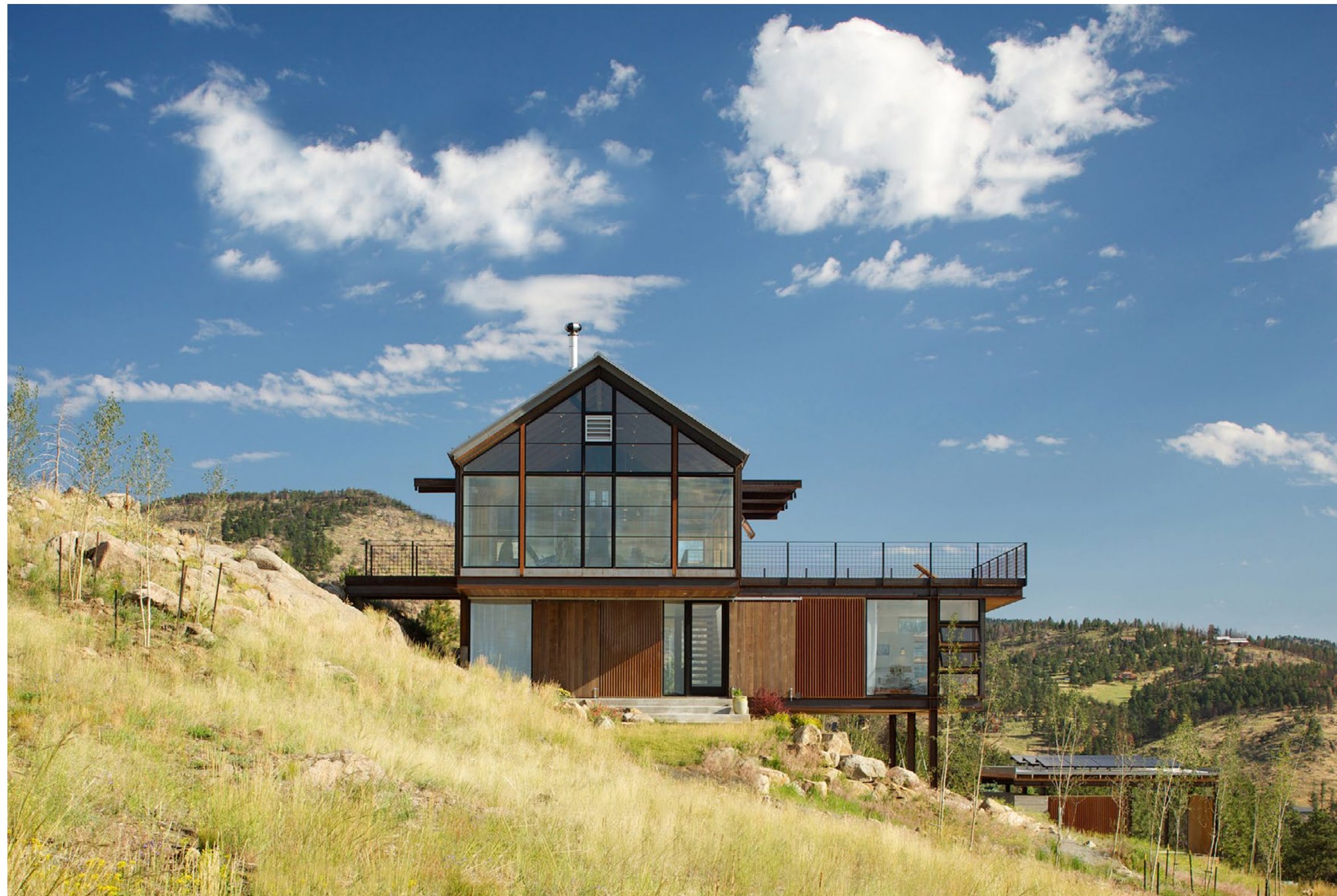
Stilt foundations to respond to sloped land
