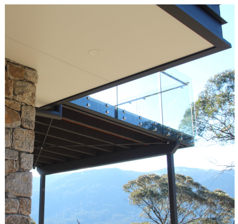
Wide overhangs for solar shading and weather protection
