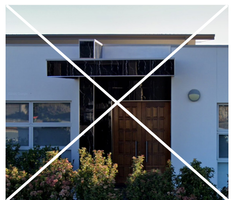
Example of inappropriate 'stuck on' tiles
