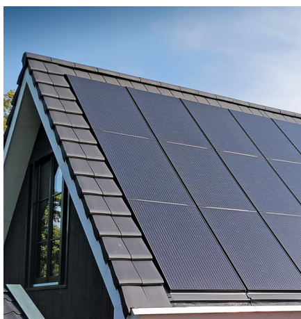
Panels to be flush with roof pitch so consider the optimal pitch, for solar value throughout the year along with external aesthetics ( sollos.com.au )
