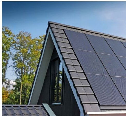
Panels to be flush with roof pitch so consider the optimal pitch, for solar value throughout the year along with external aesthetics ( sollos.com.au )
