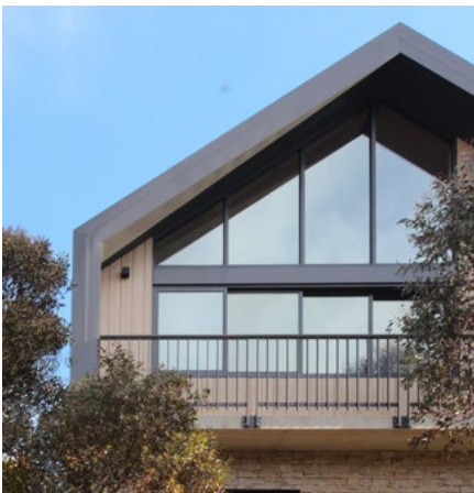
Northern view aspect facilitates solar gain through use of glazing. Wide eaves help reduce overheating in summer
