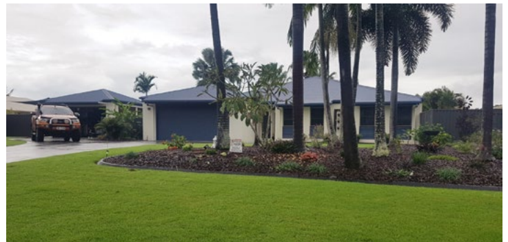
If proposing a second garage or shed to the street frontage, it must be set back from the main dwelling and complement the built-form
