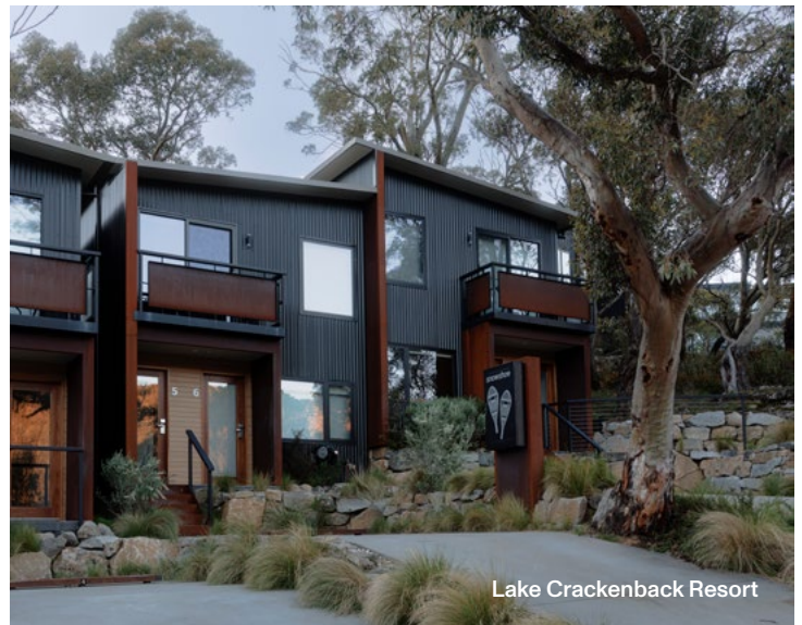
Stepped slabs to respond to the natural topography and reuse of site rock as tiered retaining wall
