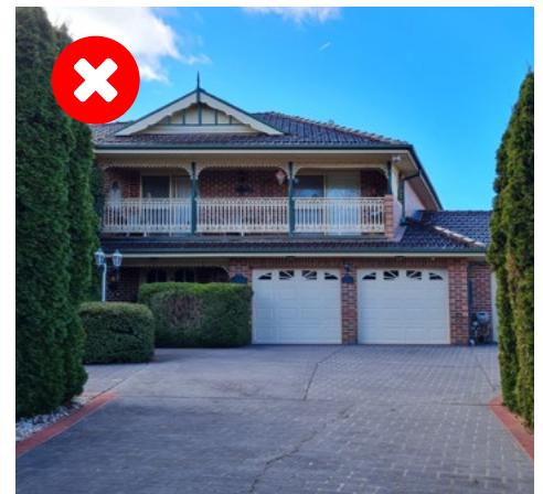
Example of replica-style architecture, inappropriate to the context and character of Mountainside
